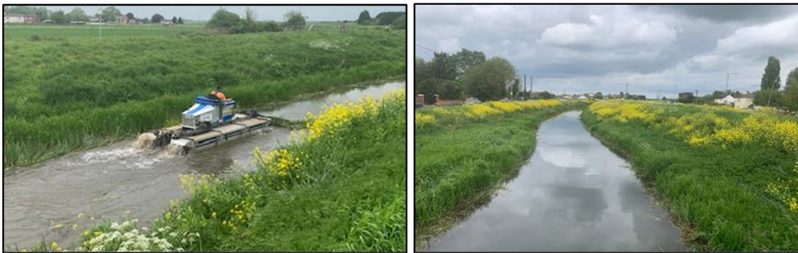
Photo 3 and 4: Weed cutting using Truxor weed boats, Billingham Skirth. Before (left), after (right)
