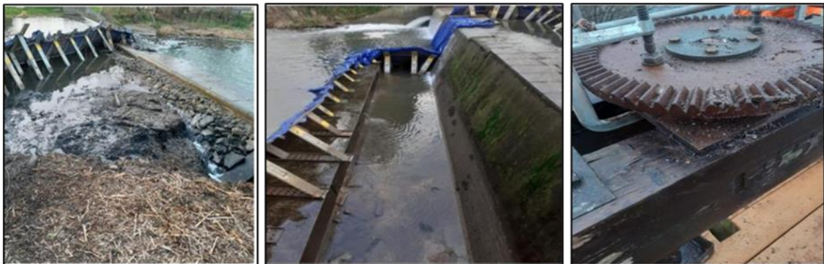
Photos 16, 17 and 18: De-watering of Claypole weir
